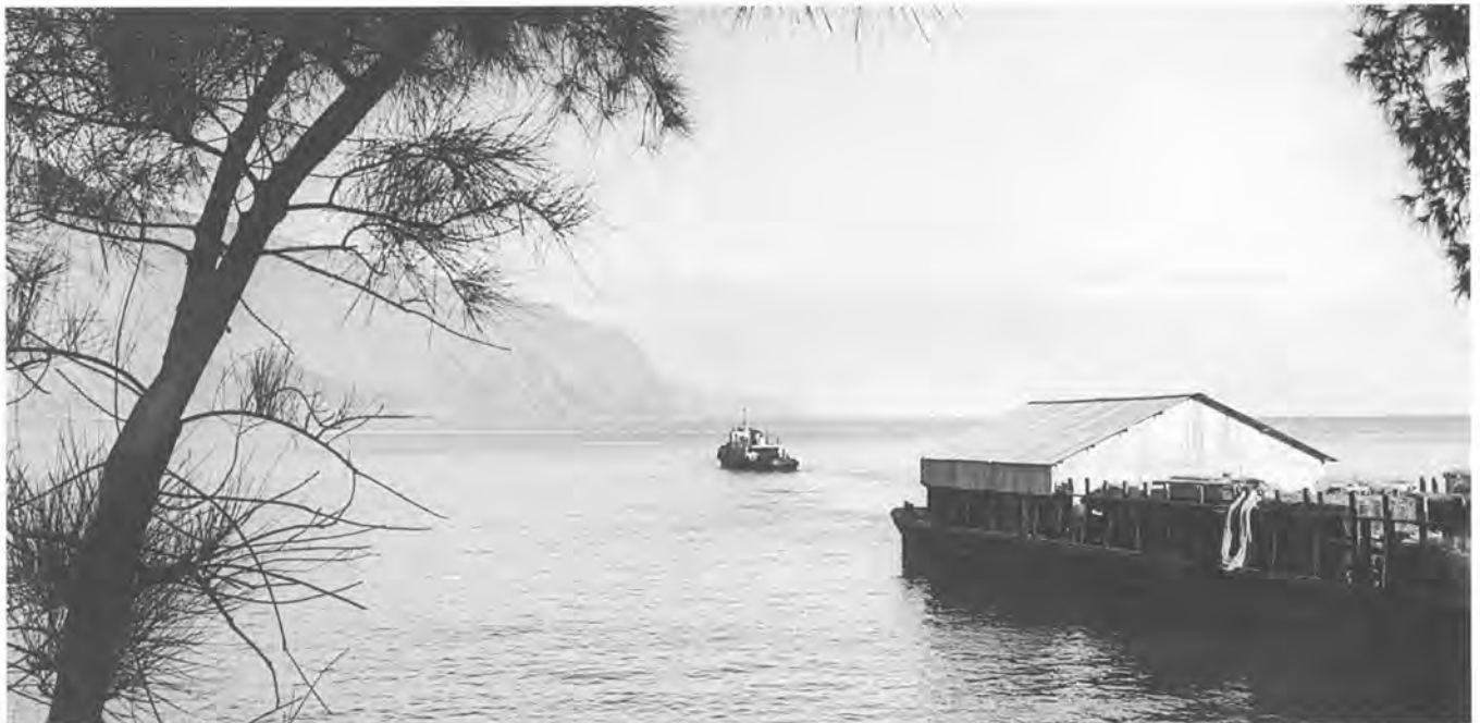
The tug Mahoe waits while a barge is unloaded at Kalaupapa. Freight barges such as this one in the 1940s carried a house to protect pallets of goods from the sea and weather.
