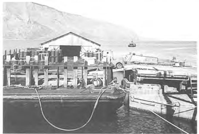
Right: Unloading a barge at Kalaupapa with oil drums carried on the open deck. An old fashioned "house" protected perishables, and a hi-lift was carried on board to move the cargo. Below: By the 1970s, the shape of the barge "house" had changed to accommodate more cargo and containers. Here, the small support tug Ma'a nudges the barge in toward the pier at Kalaupapa because the harbor is too shallow for an ocean-going tugboat.
