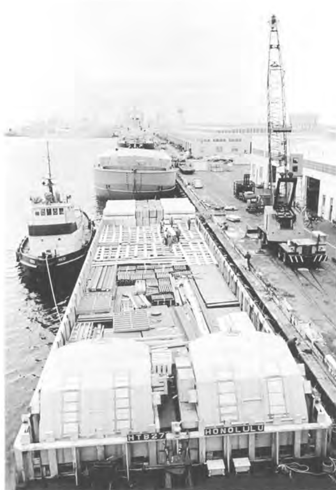
HTB-27 was used as an open deck barge that had a capacity of 1320 LT. Here the barge is being loaded with construction materials by the large crane on Pier 27. Mikioi is tied off the barge, waiting.
